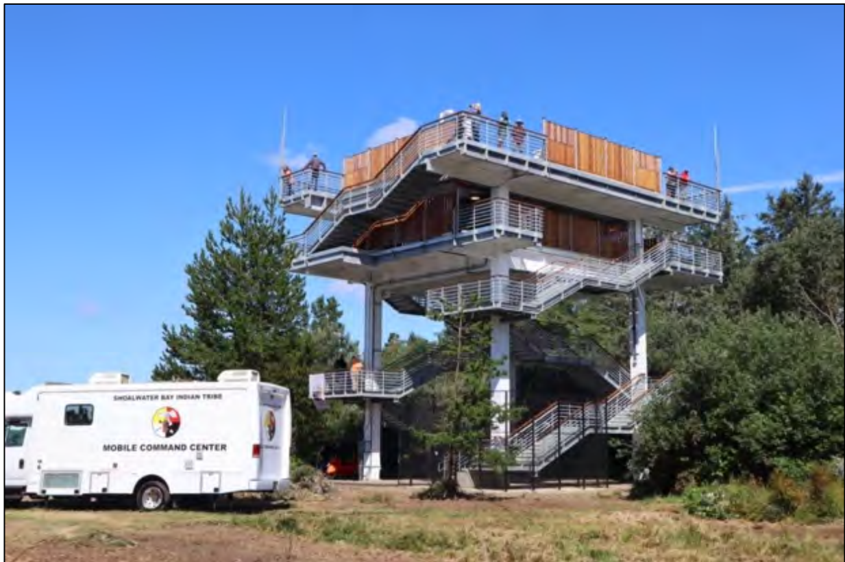
Figure 56. Tsunami Evacuation Tower. (Banse 2022)
