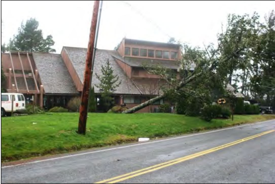
Figure 56. Tree Down on Power Line at Tribal Center, November 11, 2007.
